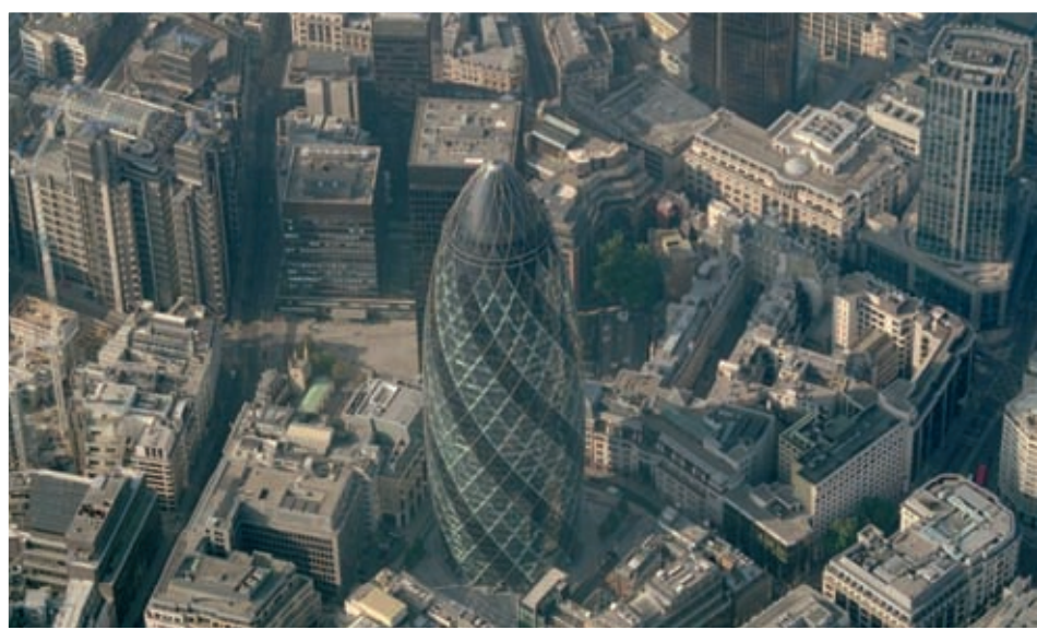
An intriguing modern office building in the centre London called the Gherkin.
