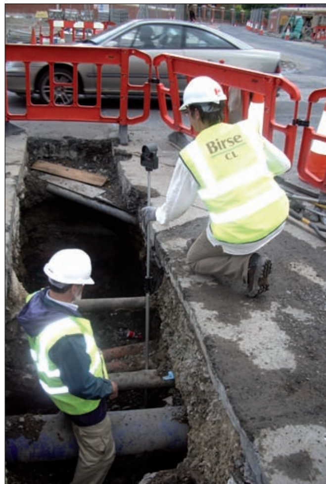
VISTA team members surveying buried utility assets.
