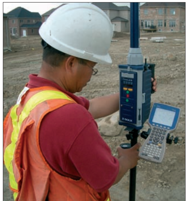
Real time surveying with Magellan Z-Max.Net corrections received via GPRS.
