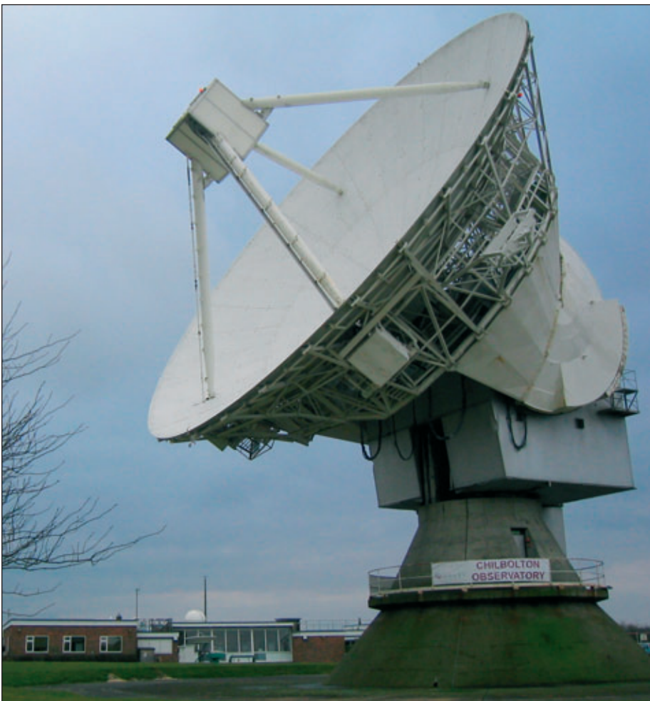
Chilbolton Observatory in England where GIOVE-A tests are being performed. (source: www.esa.int)
